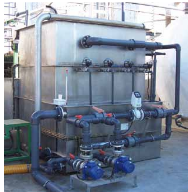
External arrangement of a MicroClear® system for wastewater treatment in the pharmaceuticals industry
